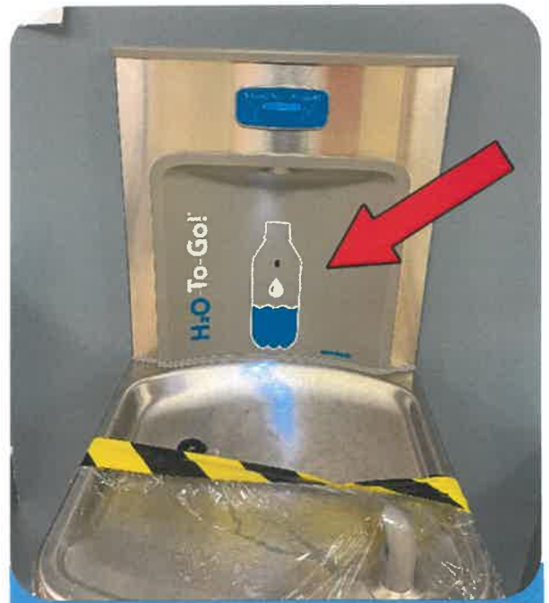
Touchless, sensor-activated bottle filler stations
