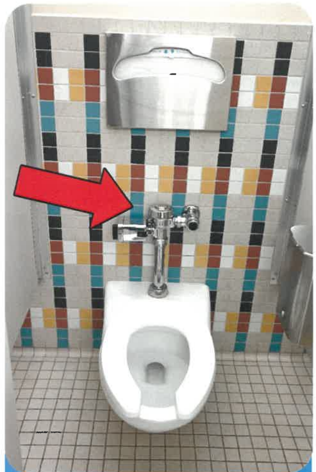
INSTALLATION OF AUTOMATIC FLUSH TOILET SENSORS IN ALL RESTROOM FACILITIES
